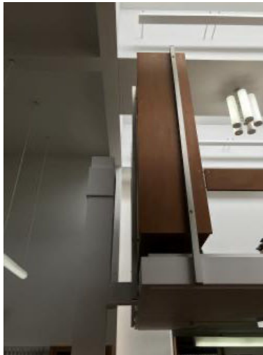
Figure 7: A close up of the mezzanine floor in the Turkish Historical Society. The non-continuity of the column and the extruded abstracted column head are visible on the left of the wood bookshelf. Source: Photograph by the author.
